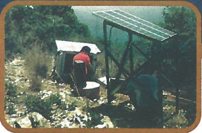
Electronic Technician giving maintenance to the station in Desecheo Island
