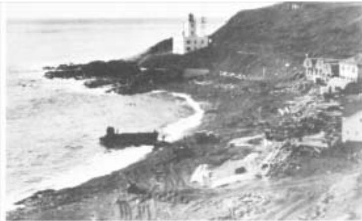
**Figure 12.36** Scotch Cap Lighthouse prior to April 1, 1946. This light is 92 feet above mean low water. Rough photogrammetric approximations result in the following elevations: foundation of lighthouse, 45 feet; foundation upper radio mast, 193 feet; upper plateau, 115 feet. [From Shepard, MacDonald, and Cox (1950).]
