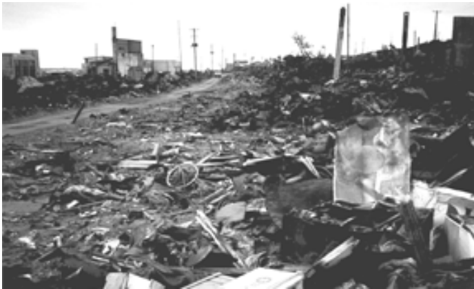
Tsunami damage at Aonae, Okushiri Island in 1993.
